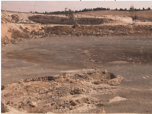
Photo 3: Wastewater pond 4B, Sep. 2019
